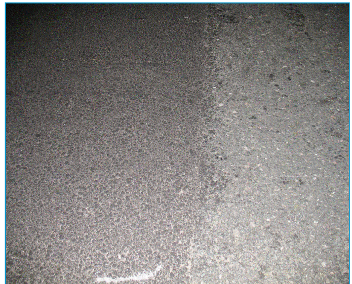
Figure 2: Close-up view before (left) and after (right) water blasting. Note the excess asphalt film thickness on the pavement surface has been removed.
