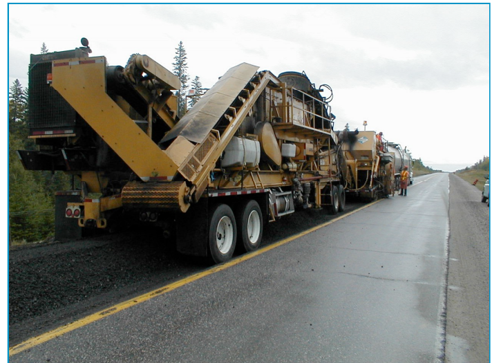
Figure 2: CIR construction train and equipment
