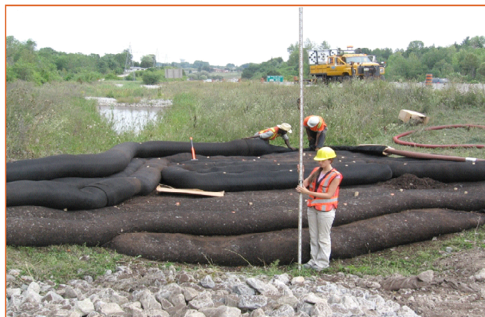
Compost Biofilter installed in the ditch on the East Side of Highway 8 near Cameo Drive, Kitchener, Ontario. Holding the survey rod is Karen Finney, a University of Guelph graduate student who led this research project.
