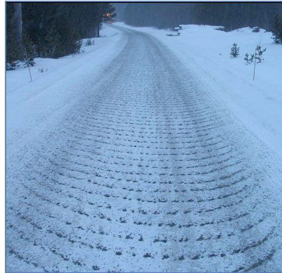
The hot water sander method is simply based on a mixture of hot water and sand.
