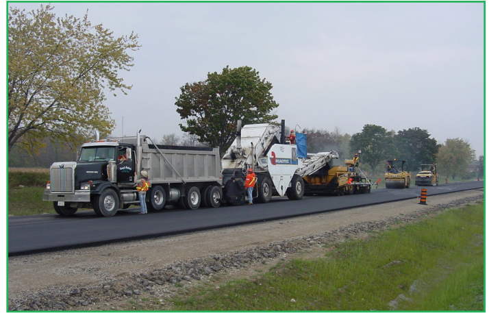
Paving on Hwy 23, West Region
