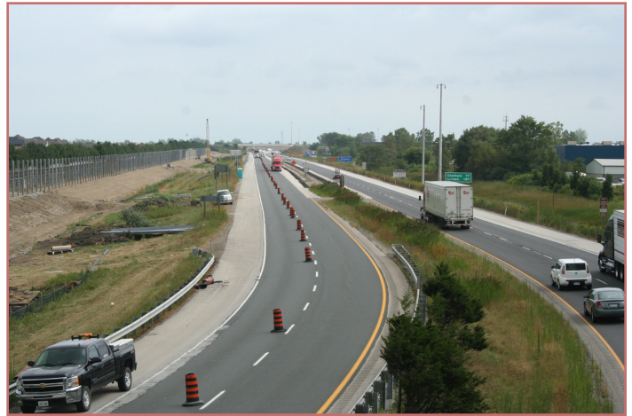
The left side of this photo shows noise barrier poles being "planted" by the highway at Tecumseh on Highway 401, in preparation for noise barrier installation.
