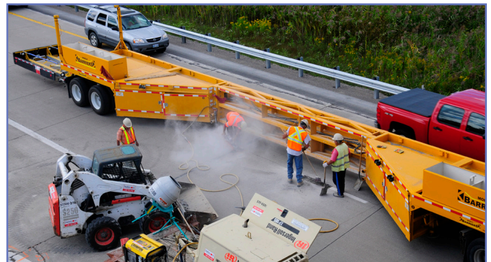
A mobile work zone barrier being moved into place for Highway 115 road work.
