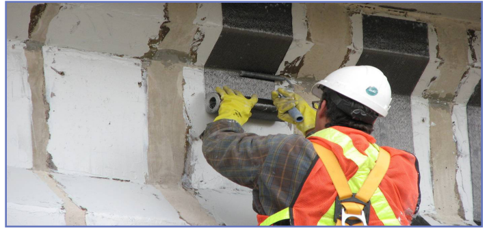
Application of CFRP strips with a roller.
