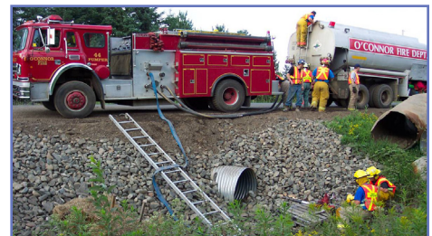
Township of O'Connor Fire Department assisted MTO in clearing the culvert with an experimental high-pressure water method.
