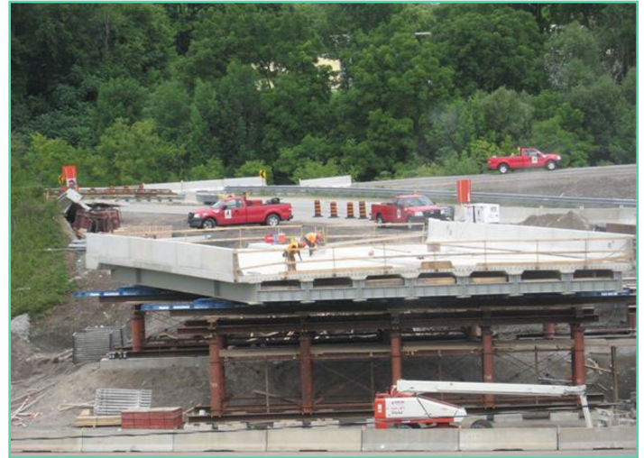
Construction of the Aberdeen Avenue Bridge over Highway 403 in Hamilton.
