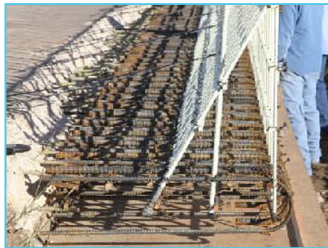
GFRP bars set up for barrier construction.
