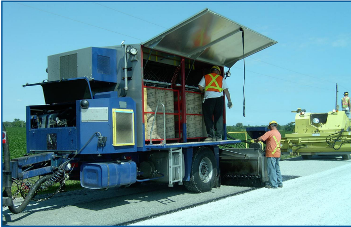
A load of 40 separate fiberglass spools capable of covering 25,000 m2.
