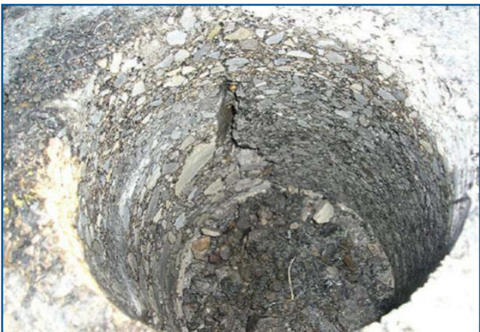
Upward crack propagation.
