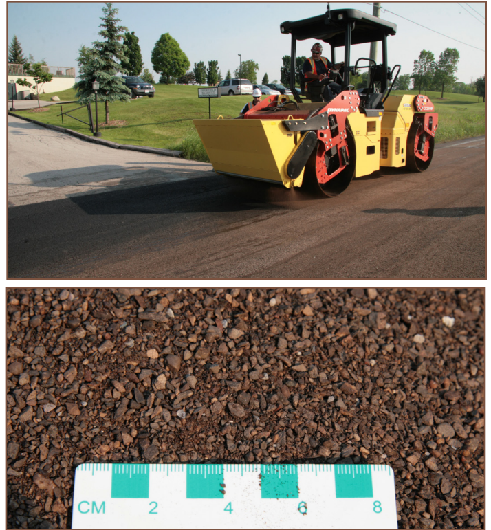
Figure 3: Gritting roller in operation at the Burlington demonstration site and close up of the loose coated grit (bottom).
