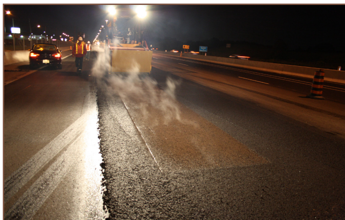
Figure 5: Coated grit being rolled in to hot SMA surface.
