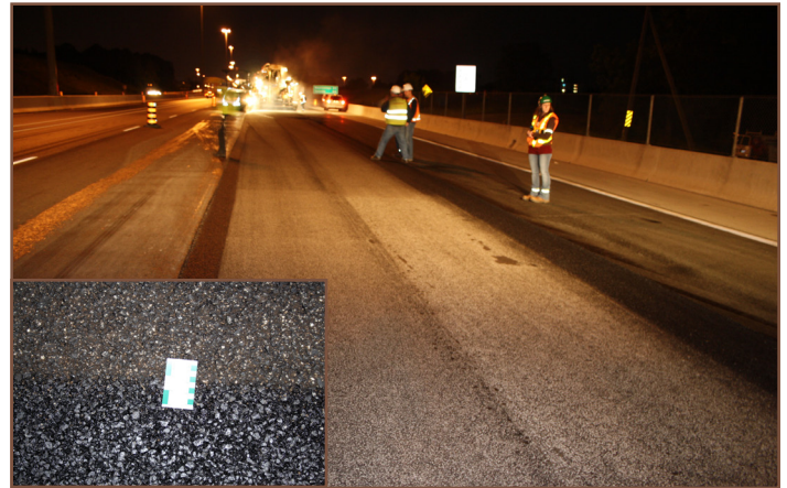
Figure 7: Texture of finished SMA surface treated with coated gritting sand and a close up (left bottom) showing differences between SMA surface textures with and without gritting.
