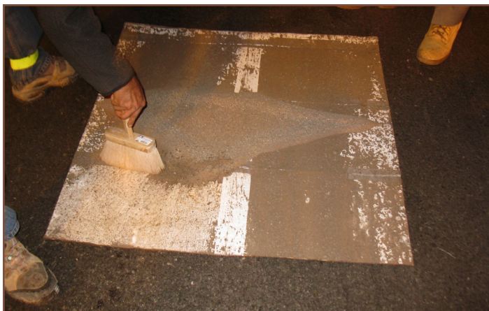
Figure 4: Verification of the application rate being carried out prior to paving. For uncoated gritting sand application, the finished SMA surface was swept to remove any excess sand (float).
