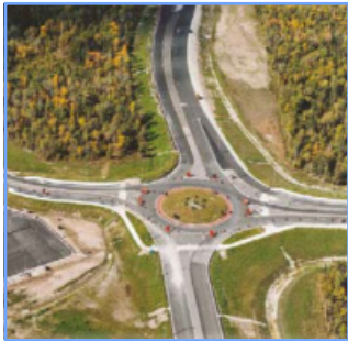
Realignment project on Highway 26, including a new roundabout.
