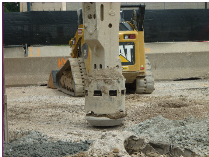
Figure 3: Bevelled tamper increases lateral pressure.
