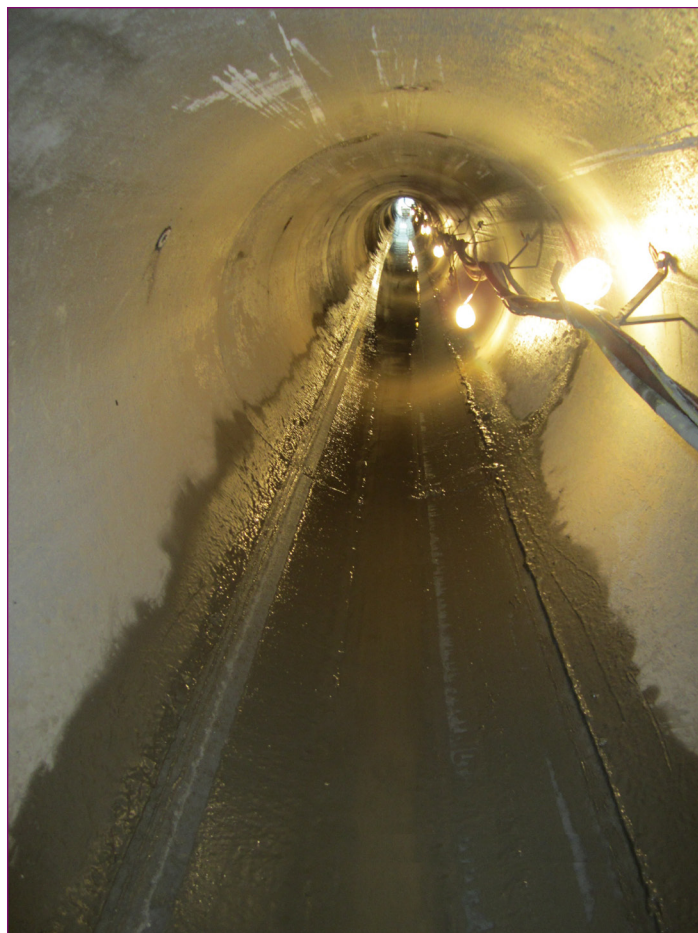
Figure 5: All concrete pipe segments installed in the tunnel.
