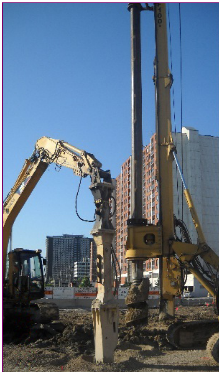
Figure 1: Rammed aggregate piers are placed within the foundation footprint of the new Canadian Border Services Agency Building in Windsor.
