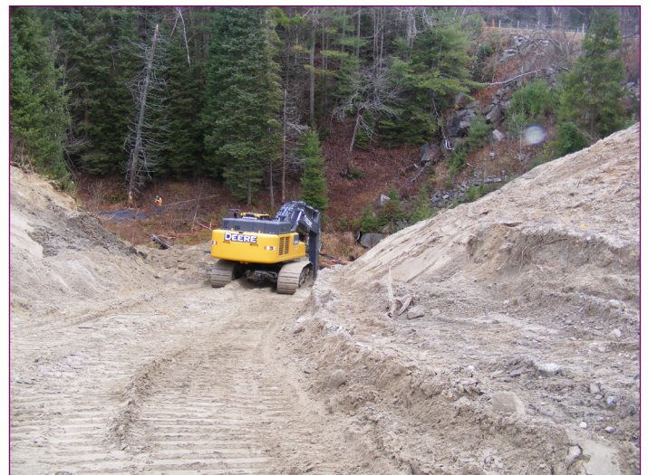
Figure 4: Access road for the exit pit located at the west side of the southbound lane.
