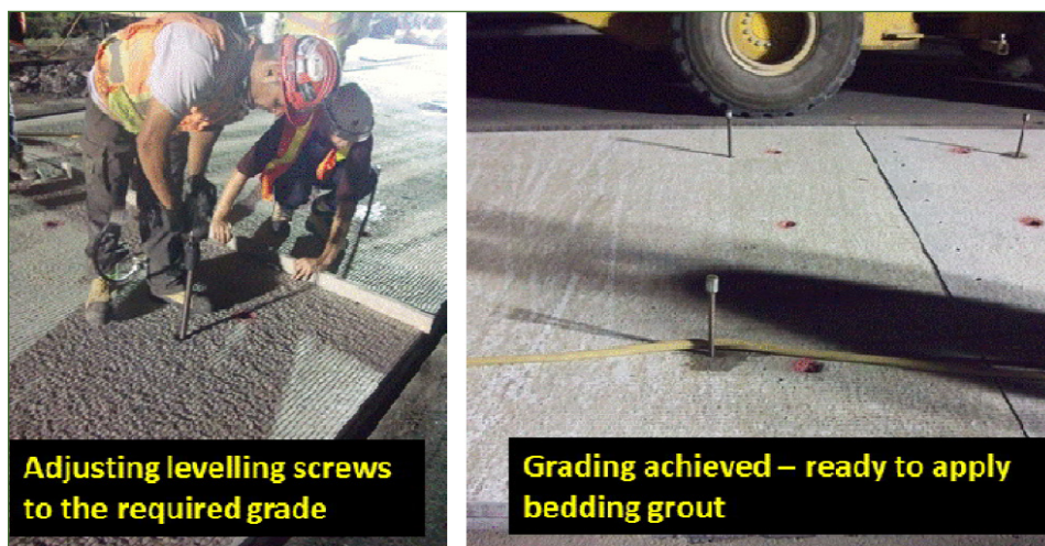
Figure 12: Grout Supported Slab Levelling Screw and Adjustment
