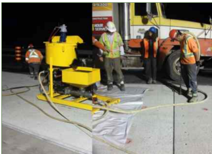
Figure 10: Pumping the Dowel Grout
