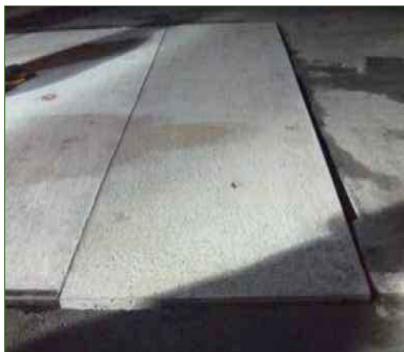
Figure 9: Asphalt Supported Slab and Temporary End Slab
