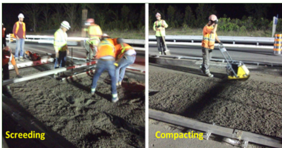
Figure 11: Compaction of the CTBM Grade Supported Slab Method
