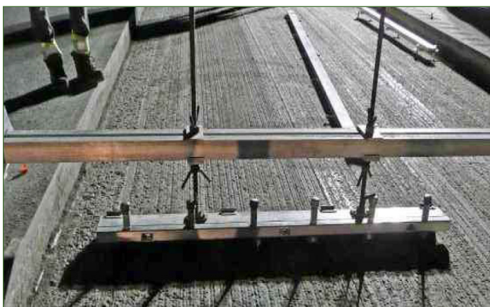
Figure 7: Fort Miller Grade Check Apparatus
