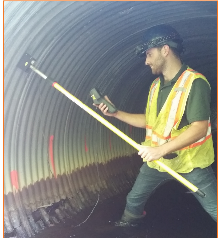
A culvert inspection technician uses the hand-held wand to identify soil voids.
