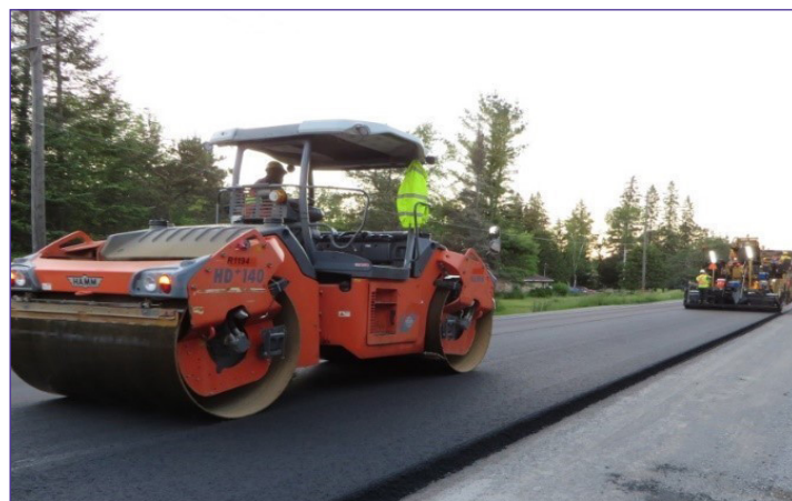
Warm Mix Asphalt paving operation showing pavement roller.
