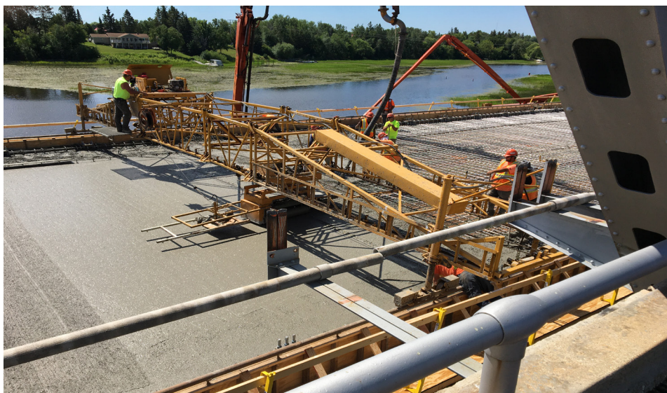
The contractor levelling concrete for the new cast-in-place bridge deck using a Bidwell screed machine.
