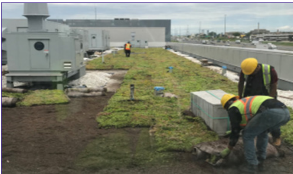
Installation of a green roof on the B-wing of the new CETI complex.
