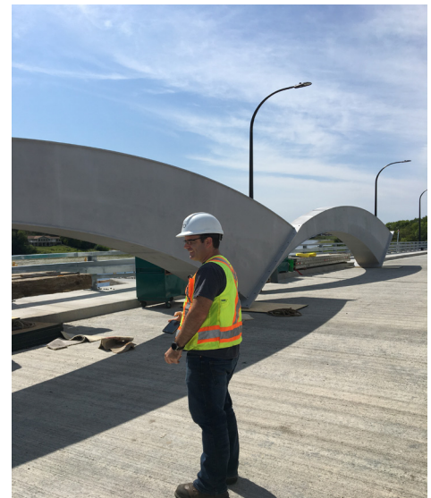
Tyler McQuaker (MTO) visually inspecting some of the arch segments prior to installation.
