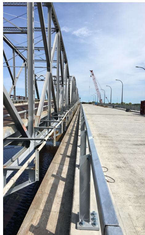
View of the narrow separation between the old bridge on the left and new bridge on the right.
