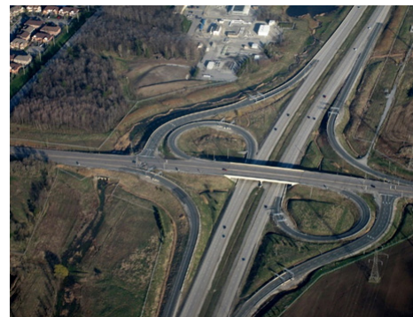
Aerial view of a partial-cloverleaf, or parclo, interchange on the Highway 407 Electronic Toll Route in Ontario
