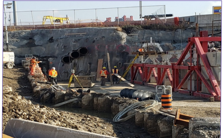
Initial set up of excavating machinery.
