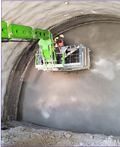
Preparing for boring phase.
