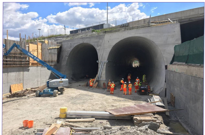
Twin tunnels and retaining walls nearing completion.
