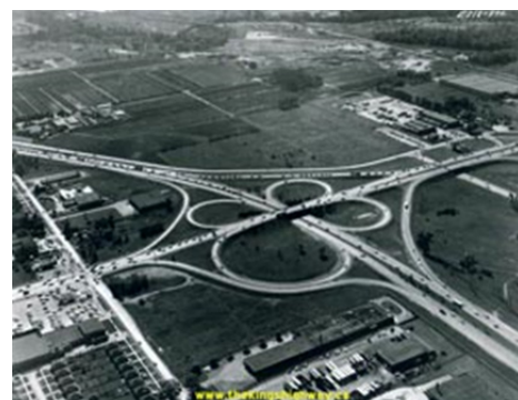
Aerial view of a clover leaf interchange on the Queen Elizabeth Way at Highway 27.
