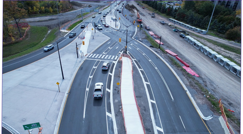
A high angle view of cars using Niagara's new Diverging Diamond Interchange.
