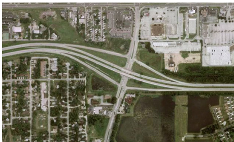
Aerial view of a typical diamond interchange.
