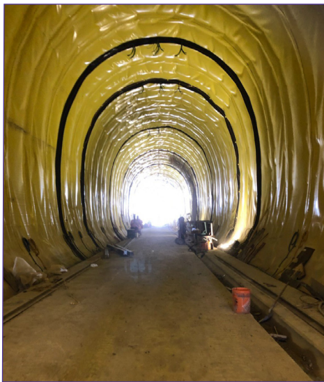
A view of the tunnel interior and waterproofing system.
