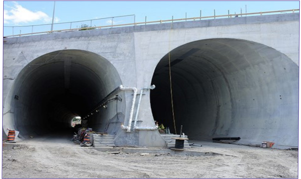
Twin Tunnels under Highways 401 and 409.
