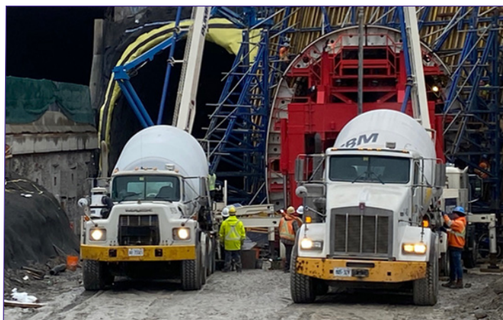
The new twin tunnels beside the existing tunnel.
