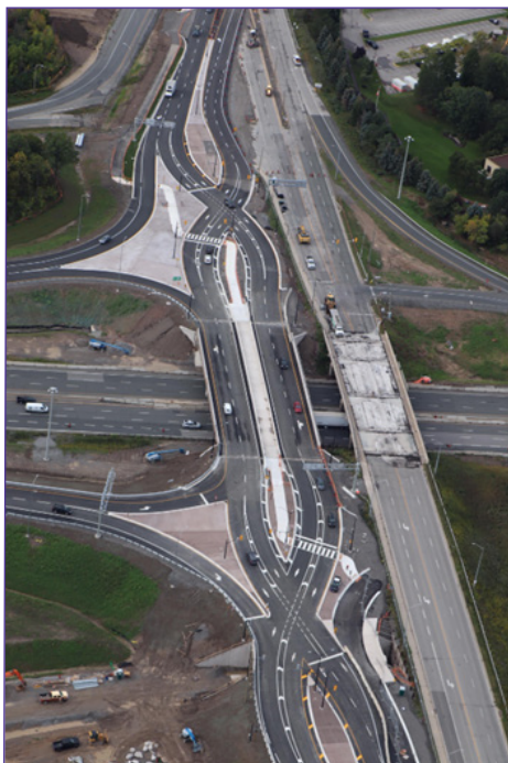
Aerial view of the new Diverging Diamond Interchange in Niagara.
