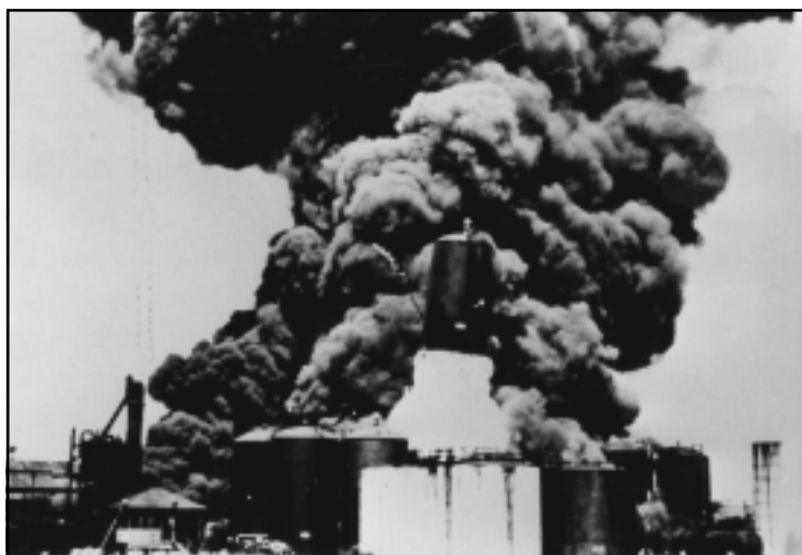
ROCKET: Inadequate emergency relief venting can cause tanks to explode violently or rocket great distances.*
