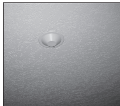
A picture of how the finished product looks in all the ceilings. If a fire were to occur, the cap on the sprinkler head would separate at 135°F and allow the sprinkler head to activate at 155°F.
