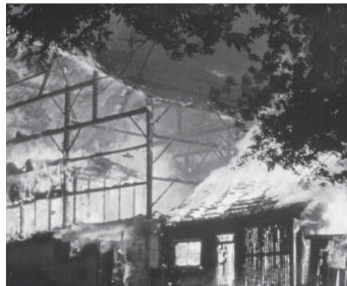
Historic barn on fire. Picture courtesy of John Johnson.
