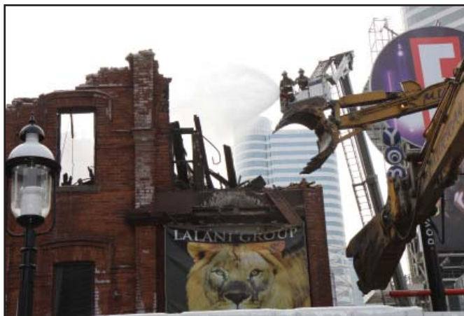
A picture of the demolition efforts at Yonge and Gould Streets in Toronto to tear down a historic building. The first day, Toronto Fire Services firefighters were on stand-by to extinguish any remaining hot spots.
