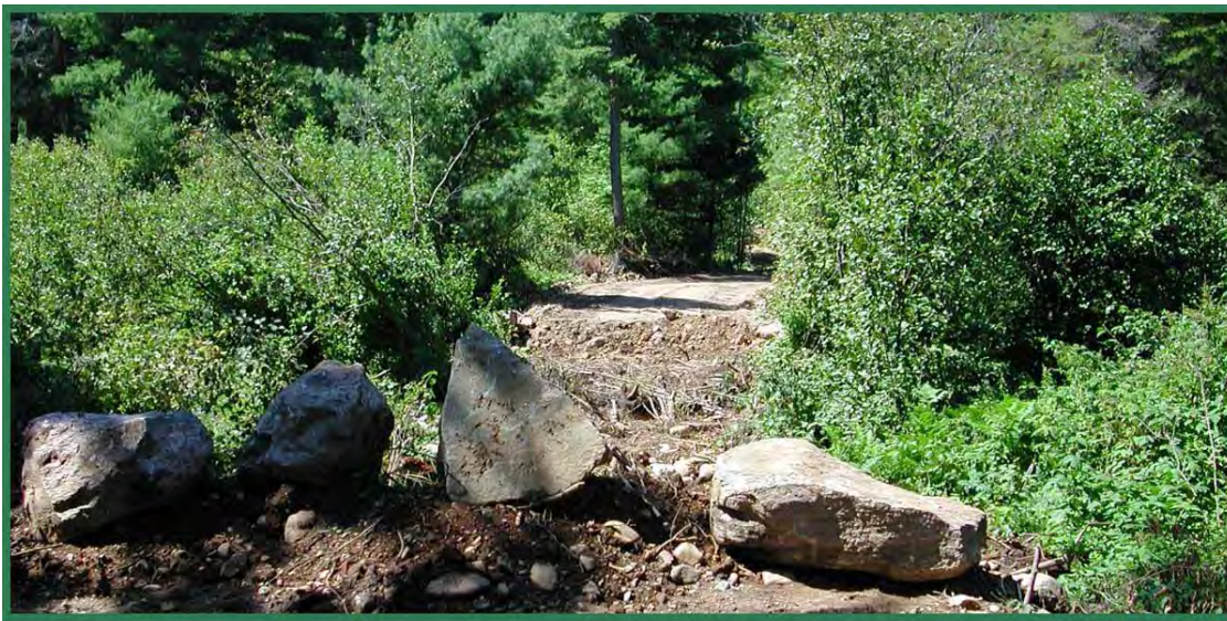
Physical road decommissioning
