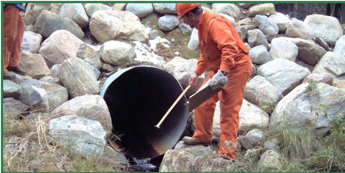
Culvert Inspection (road and water crossing compliance activity)
