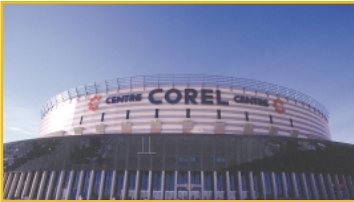
Ideal Roofing supplied 136,078 kilos of siding for the interior and exterior walls of the Corel Centre in Ottawa.
