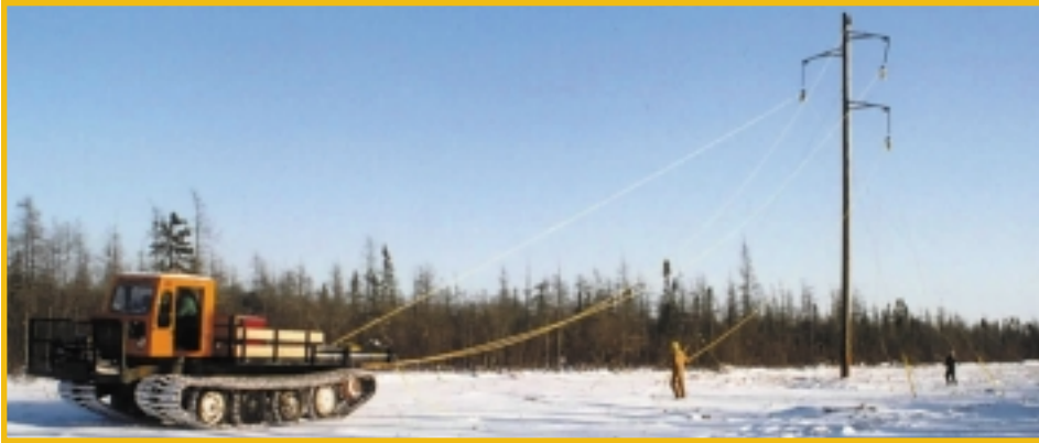
A crew works to “string” transmission lines that will bring electrical power to remote Northern Ontario communities.
