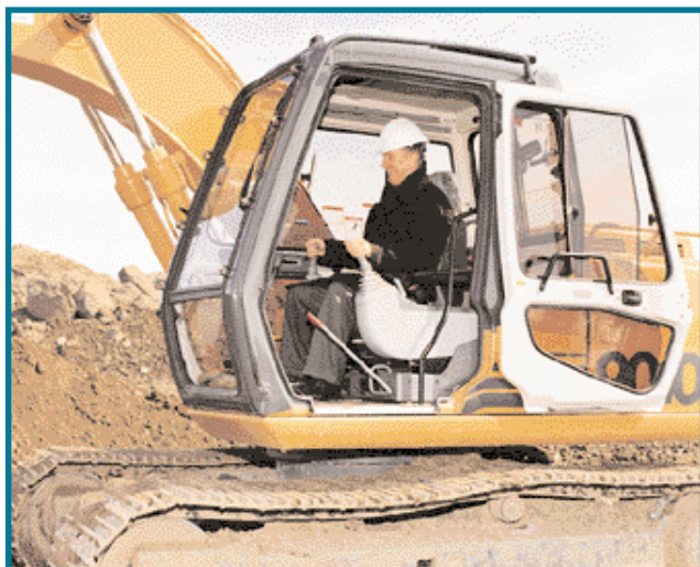
MEDT Minister, Bob Runciman operates a large excavator at OETI event held in March.
