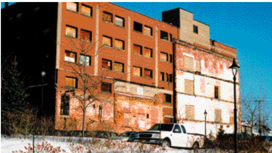
Part of this building on the Cornwall PDF project site will be redeveloped into model residential units.
