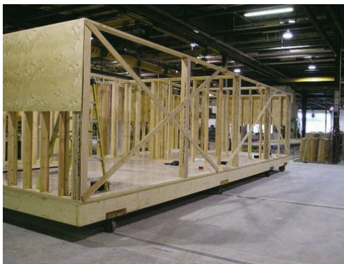
All Royal Homes are built indoors in sections which are assembled on-site. Everything from interior finishing to electrical, plumbing and flooring is installed before the house is transported to the foundation.
