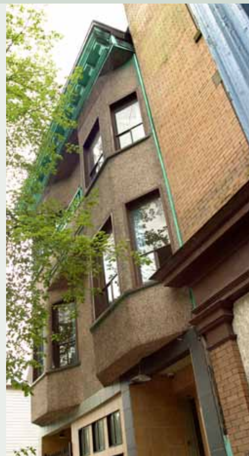
The Vivian is the first minimal barrier housing program in Vancouver for women with complex needs.
