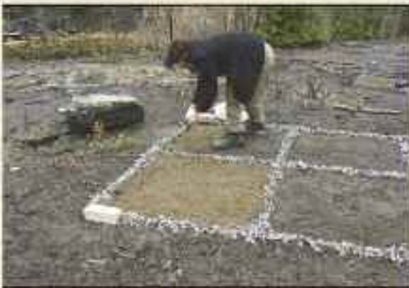
(a) laying down sand substrate amendment.
