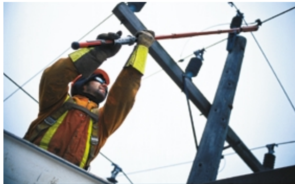
Wood pole replacement / Allanburg
