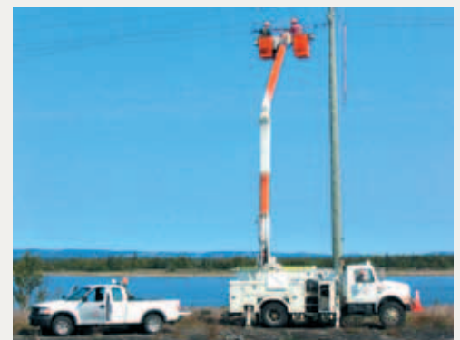
Crews string new lines to improve reliability on Manitoulin Island.
