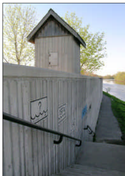
Part of the flood protection works in Cambridge, showing a water level gauge station and plaques marking the height of previous floods.
