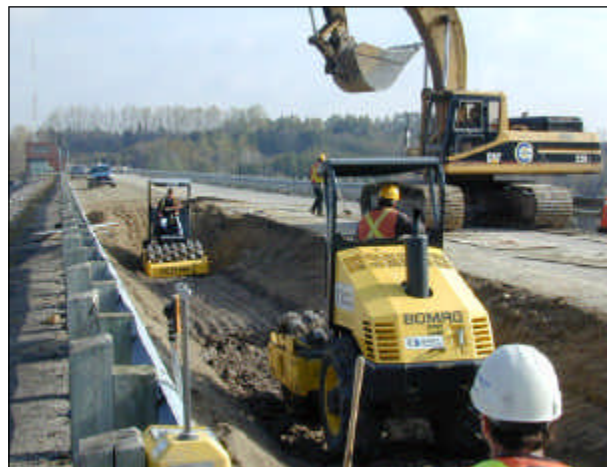
About $1.4 million was invested in dams and dikes.
