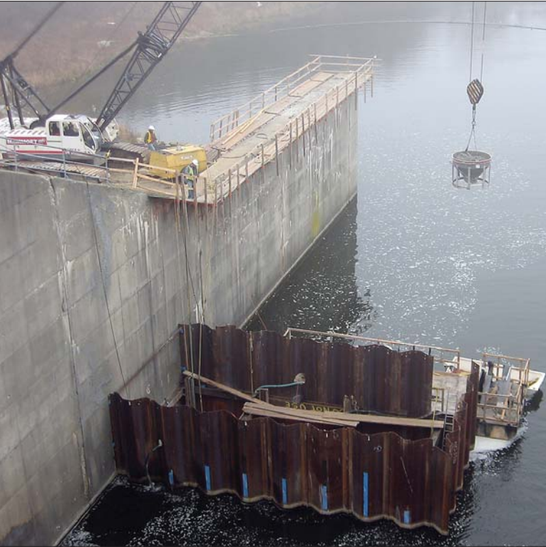
A load of cement is lowered into place during a $2.7 million upgrade to the Conestogo Dam stilling basin that will allow it to safely handle higher flows.
