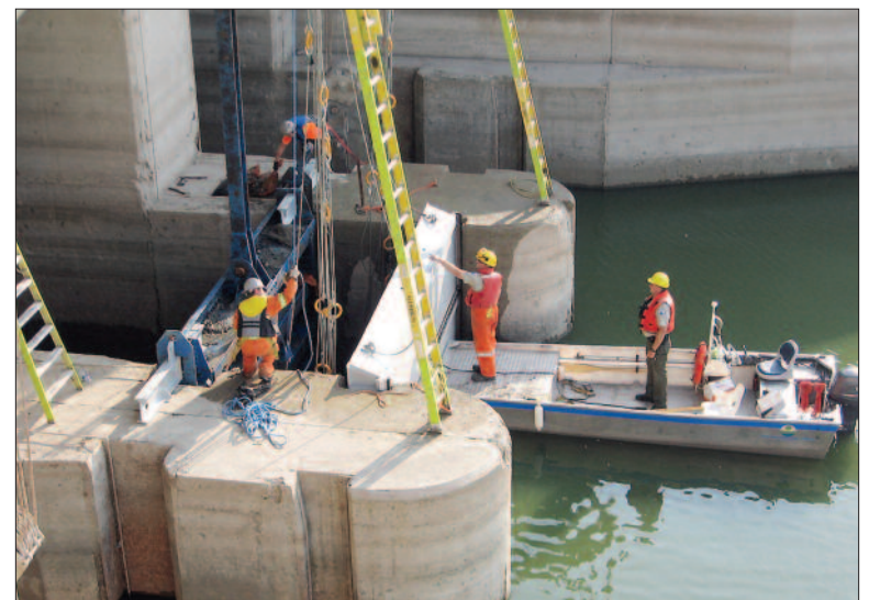
The Conestogo Dam gates were refurbished in 2012 for $84,000. The dam reduces flood damages and maintains river flows in the summer.
