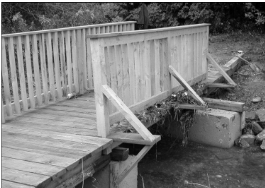
A four metre (13 foot) walking bridge was made by Trees Unlimited in Welland, and Townsend Lumber in Tillsonburg and "won" by The Grand River Foundation at Canada's Outdoor Farm Show in September. Cambridge volunteers placed it at the Dumfries Conservation Area, where it will make this natural area more accessible to hikers and nature lovers.
