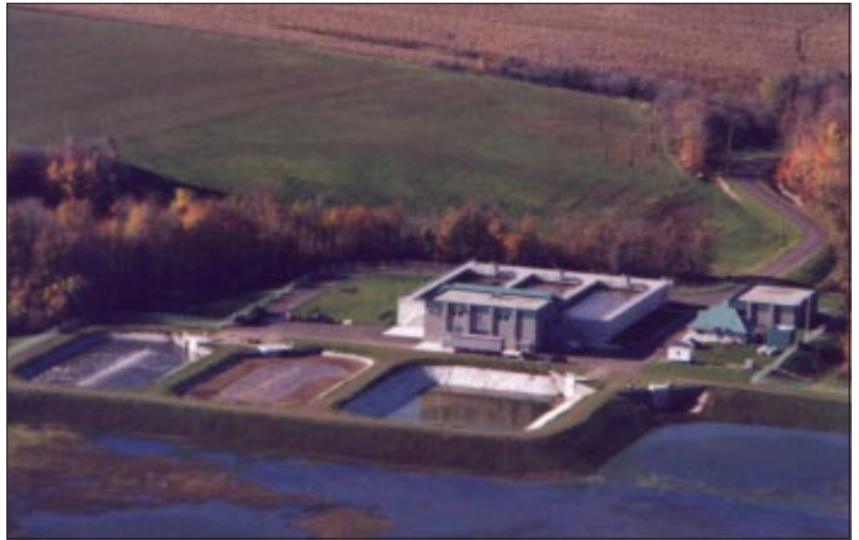
This aerial photo of the newly opened New Hamburg Wastewater Treatment Plant shows the state of the art plant and the emergency lagoon which has been retained for temporary storage during unusually heavy rainfall.
