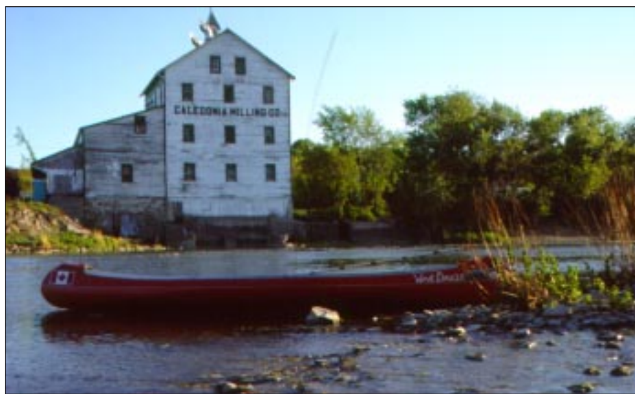
Caledonia Mill represents part of the industrial heritage of the southern Grand River. The river also plays a major role in the recreation of many watershed residents. The mill has recently been restored. Photo: Daryl Baxter.
