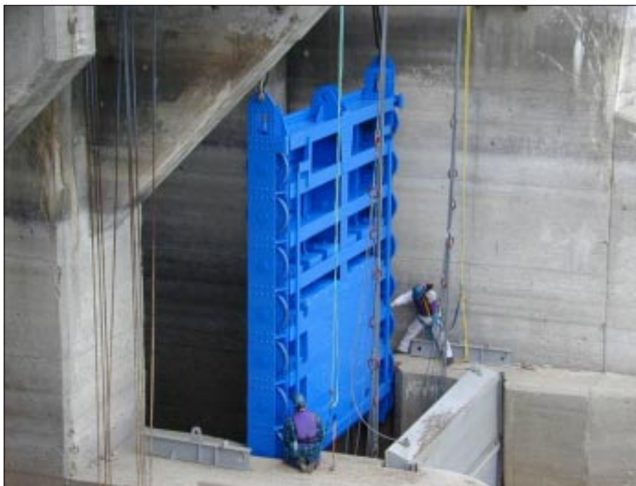
Conestogo Dam gates get much needed repairs over a two year period. This photo shows workmen installing one of the repaired gates at the dam.
