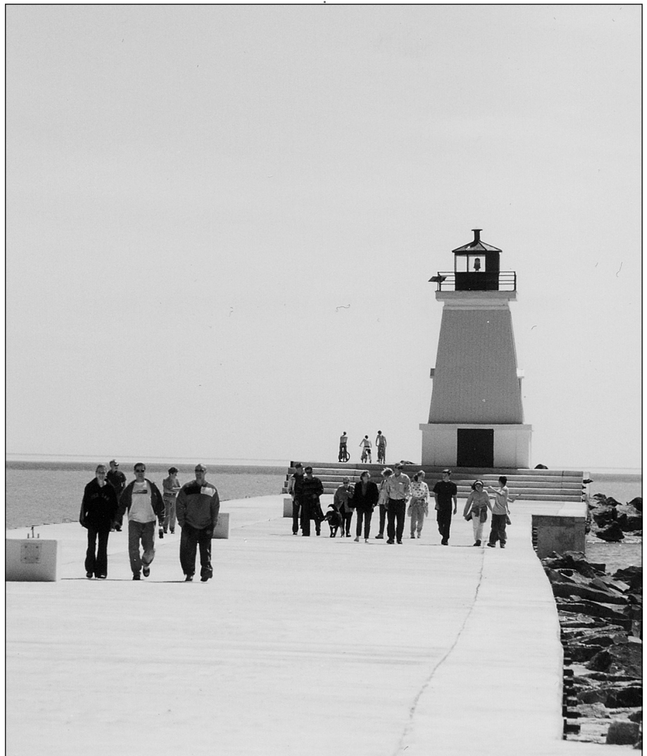
The west pier in Port Maitland, at the mouth of the Grand River, has been rebuilt and the lighthouse refurbished as part of a $5 million project of the federal government.
