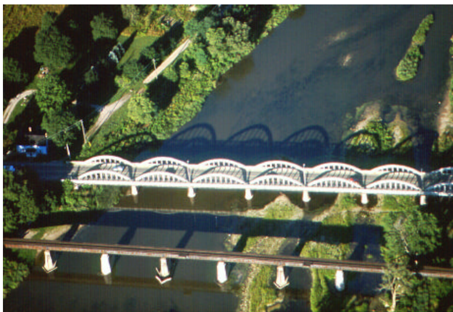
The Freeport Bridge in Kitchener, currently being refurbished, is one of several historic bowstring bridges spanning the Grand River. (Photo by Carl Hiebert)
