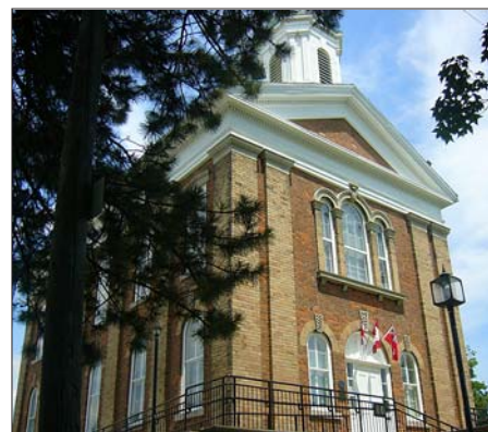
Caledonia Town Hall is on the Creepy Caledonia tours that will be taking place this summer and fall to raise funds for the Caledonia Agricultural Society.
