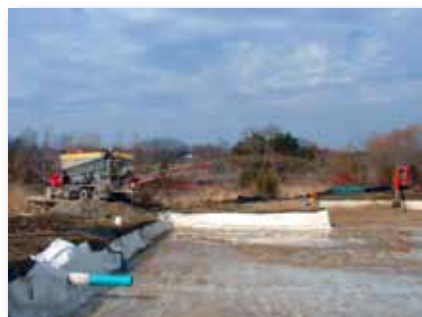
Installation of red sand filter
