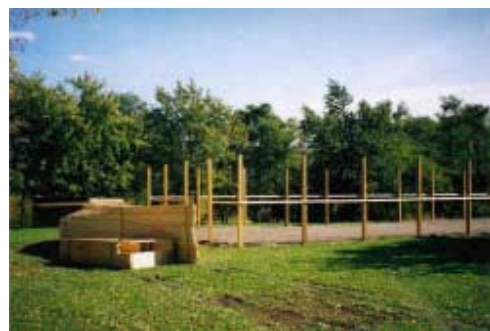
A large pavilion is being constructed by the Wheatley Two Creeks Association at the Two Creeks Conservation Area. It is located in the south end of the park.
