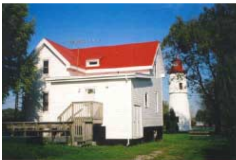
The restorations to the residence and Lighthouse structure located at Lighthouse Conservation Area were completed this fall.
