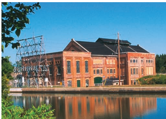
Healey Falls Generating Station
