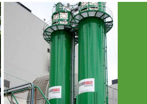
▲ Biomass storage silos - Nanticoke GS
