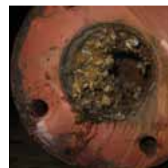
▲ Cross-section view of water pipe blocked by mussels.
