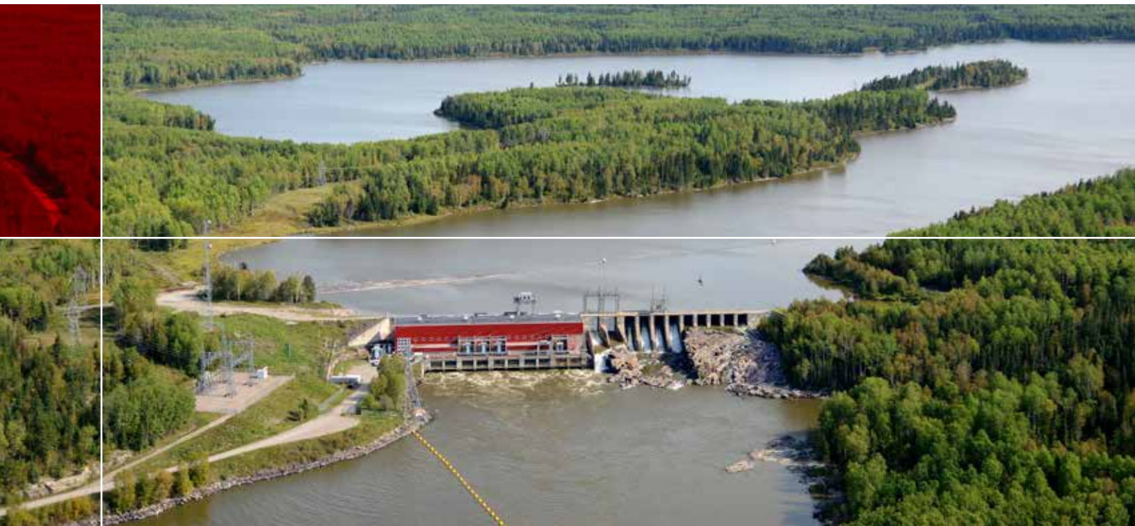
Manitou Falls Generating Station
