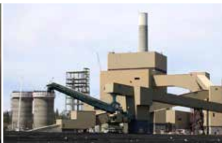
Atikokan GS biomass conveyor and storage silos
