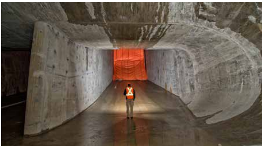
An OPG employee examines the concrete draft tubes of Smoky Falls Generating Station.
