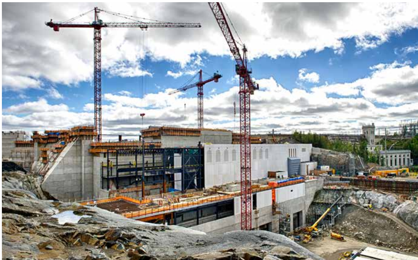
Construction at the Smoky Falls Generating Station
