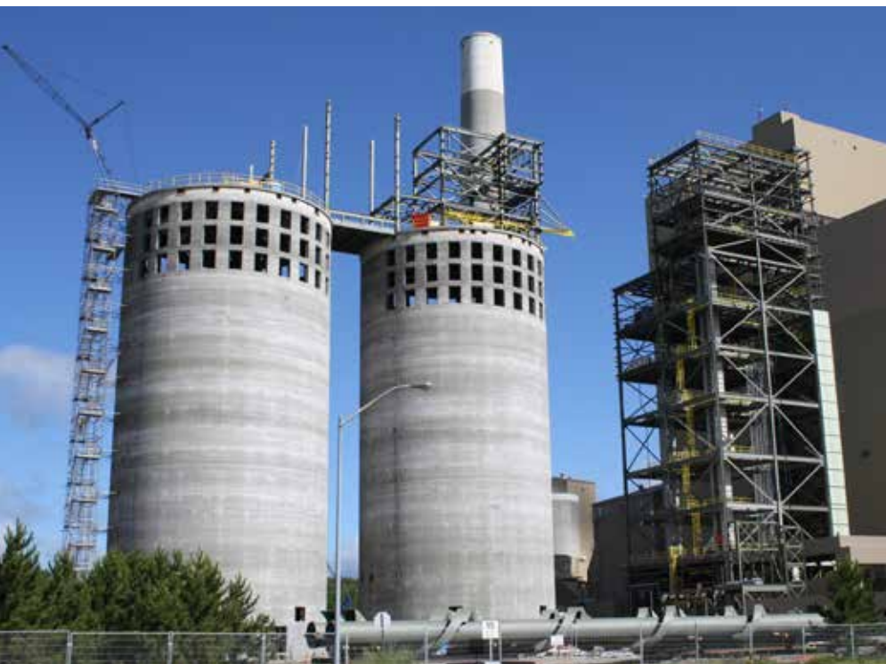
Biomass storage silos at Atikokan Generating Station.
