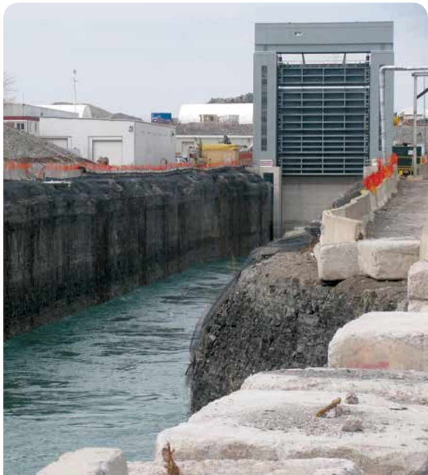
New Niagara Tunnel outlet tunnel and gate
