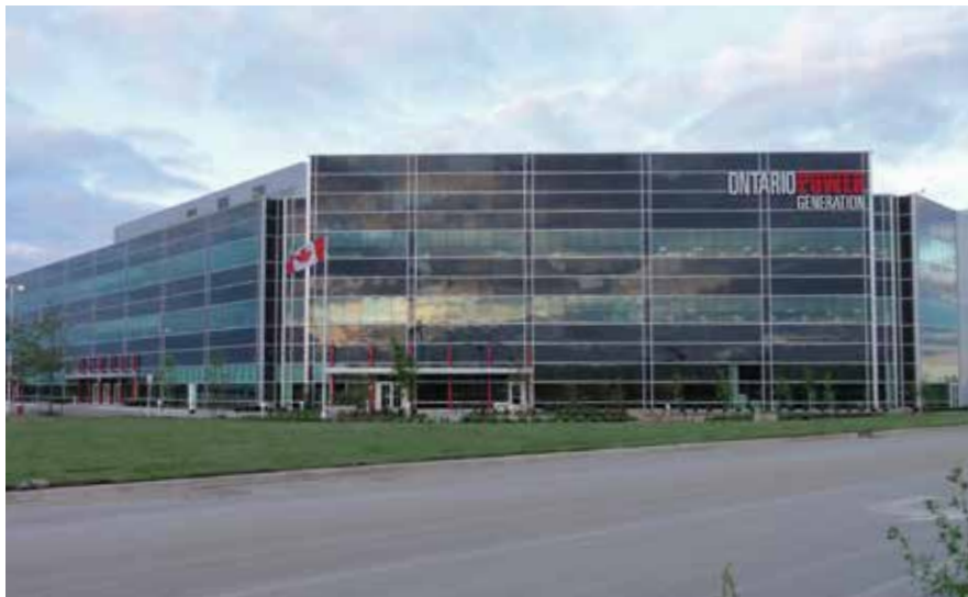
Darlington Energy Complex located in Courtice, Ontario.
