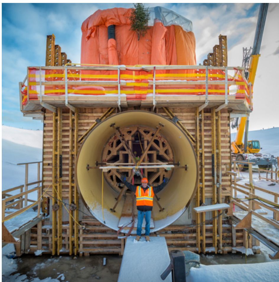
Construction of the Peter Sutherland Sr. GS.
