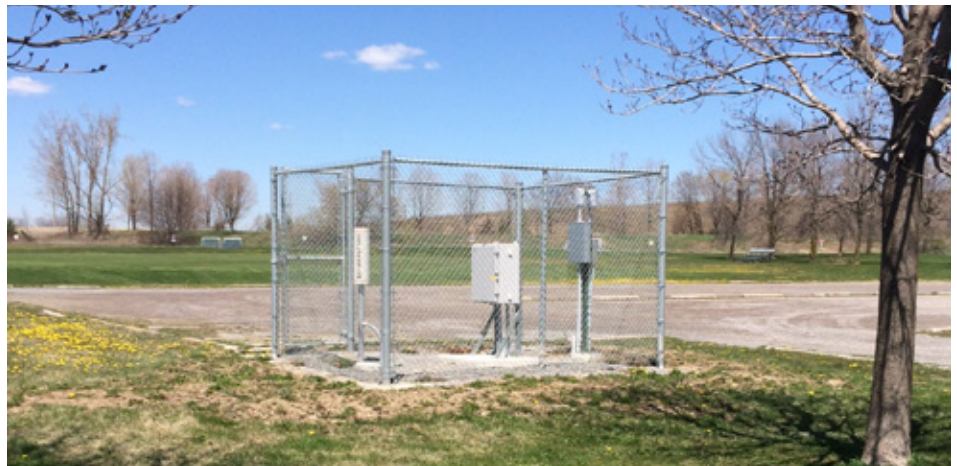
Environmental monitoring station.
