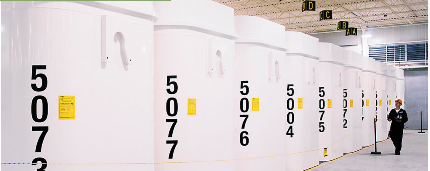
Used nuclear fuel storage containers.
