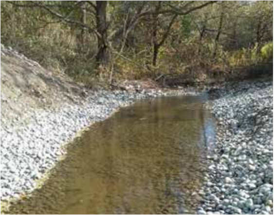
Left: Creek restoration at the Wesleyville site.
