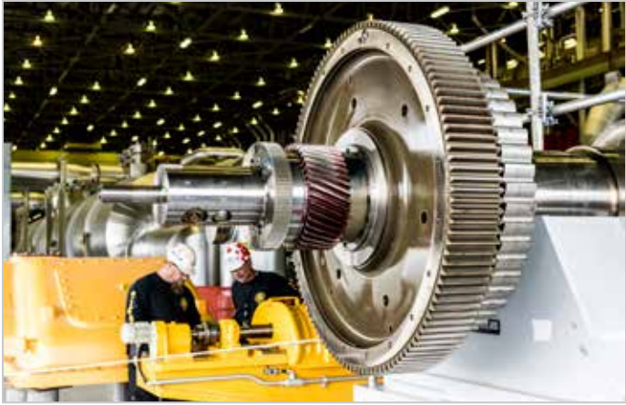
OPG and its partners are working to complete the Darlington Refurbishment safely, on time and on budget.
