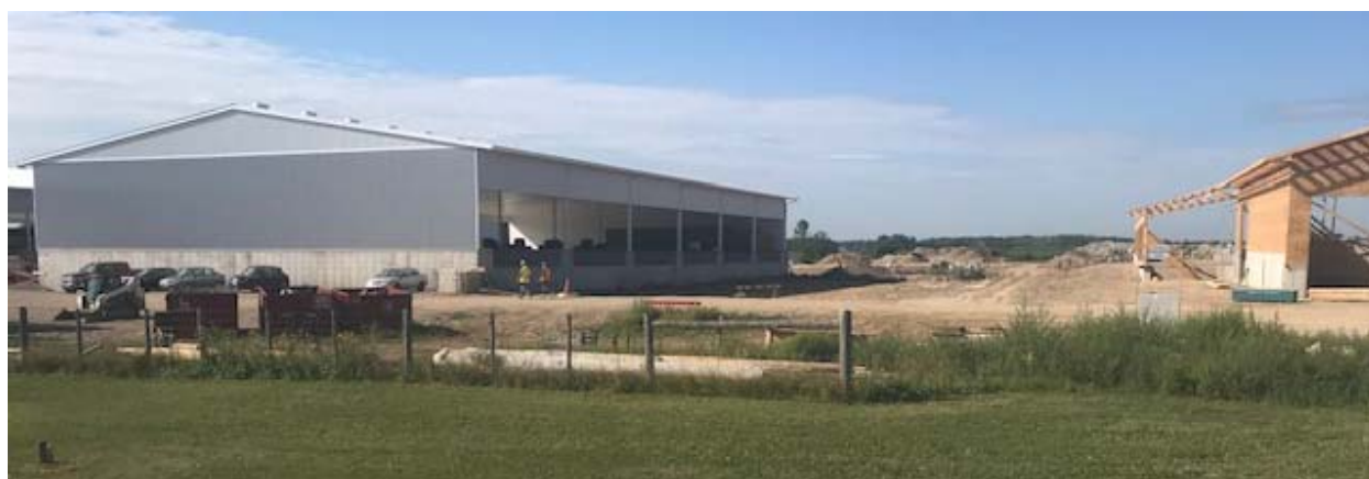
Figure 2: Elora feed storage being constructed.
